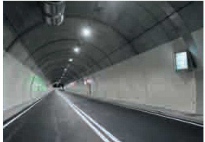
Blick in den Tunnel - 16.4.2011 (Foto: Perfl)
